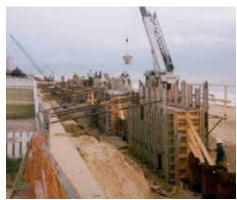
sheet piles (28-foot lengths) supplied by Nucor Skyline. The main wall is cantilevered in some sections, and in others, anchored to a secondary wall of Z-shaped sheet pile. According to Roehrs, the design would protect against a 9-foot surge and "survive a 1-in-146-year storm."
